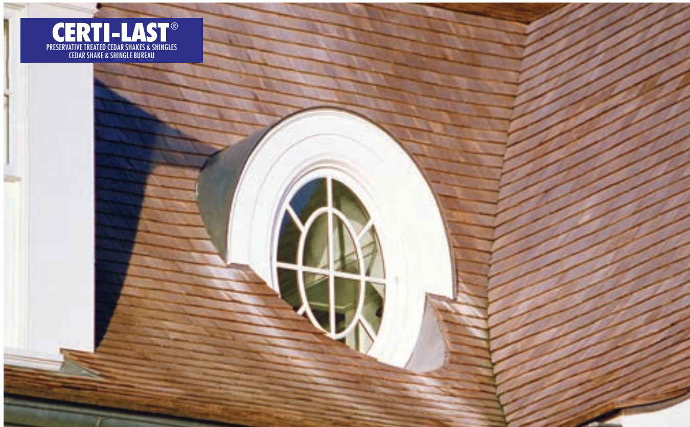
Courtesy: C&H Roofing Inc.
