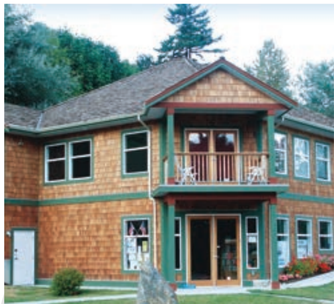
Photo below shows Certi-label® Western Red Cedar installation
