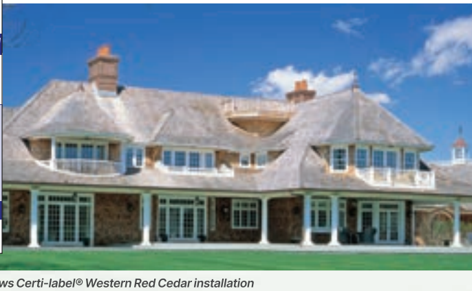
Photo Shows Certi-label® Western Red Cedar installation
