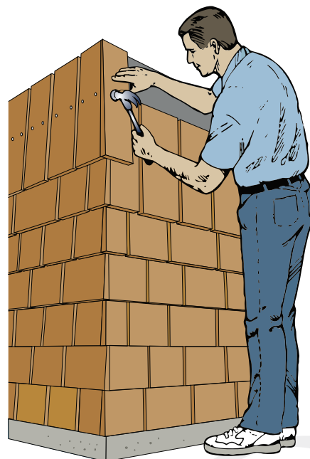
Figure 9: Fitting Laced Corner Courses
