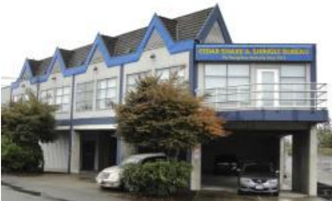
The Cedar Shake and Shingle Bureau office in Mission, BC. This is where the archival research and organization was performed.
