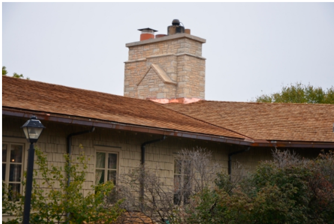
The finished installation. Note copper flashing and completely rebuilt chimney.
