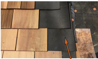
Rot felting of tapersawn shakes
