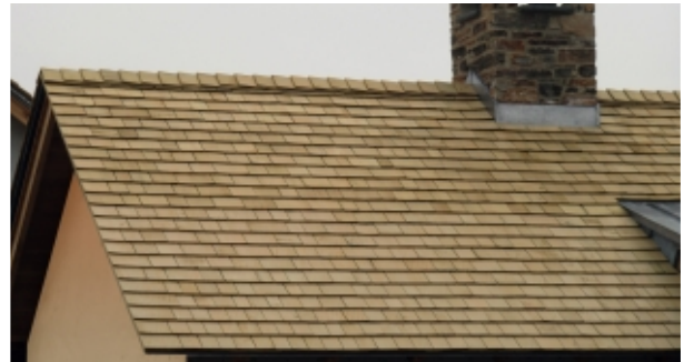
A finished Certi-Sawn® yellow cedar tapersawn shake roof
