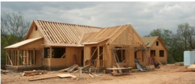
Framing work is well underway
