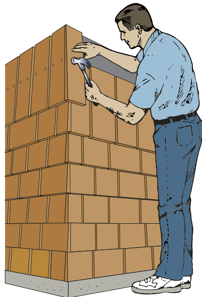
Figure 9: Fitting Laced Corner Courses
