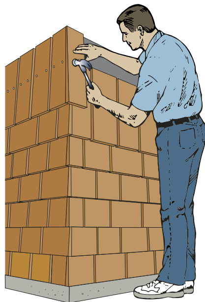
Figure 9: Fitting Laced Corner Courses
