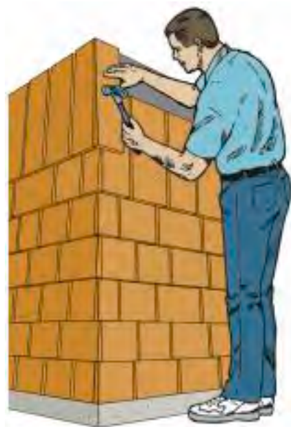
Figure 9: Fitting Laced Corner Courses
