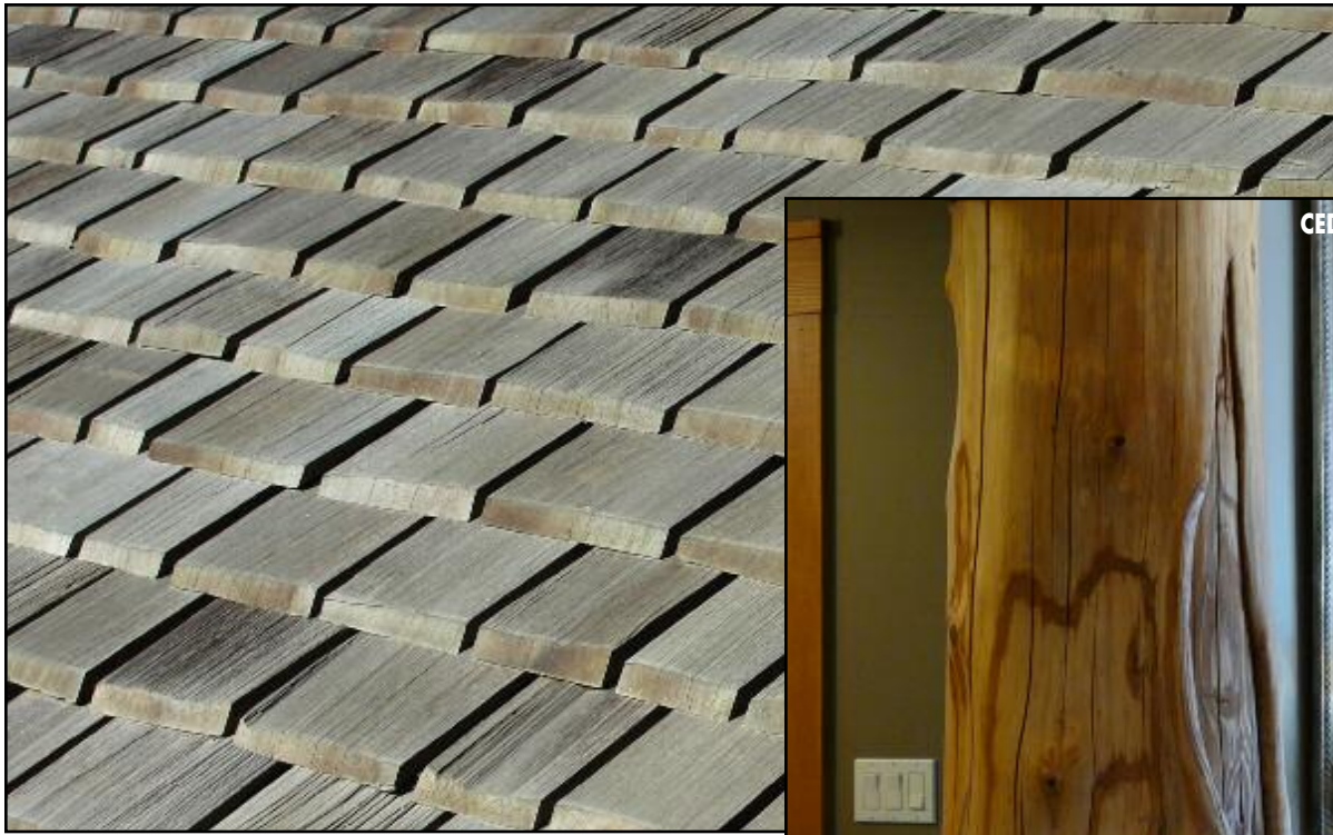
1 INCH THICK WESTERN RED CEDAR SHAKES WITH BEVELED BUTTS WHERE USED ON THE ROOF.
