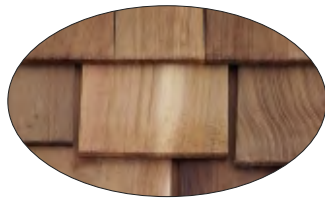
Uneven courses (on non-staggered butt roof)
