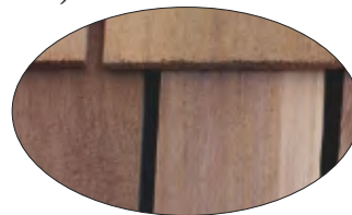
Exposed interlaid felt
