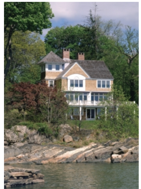
Brindisi and Yaroscak Custom Builders, Inc. Architect: George Dumitru
