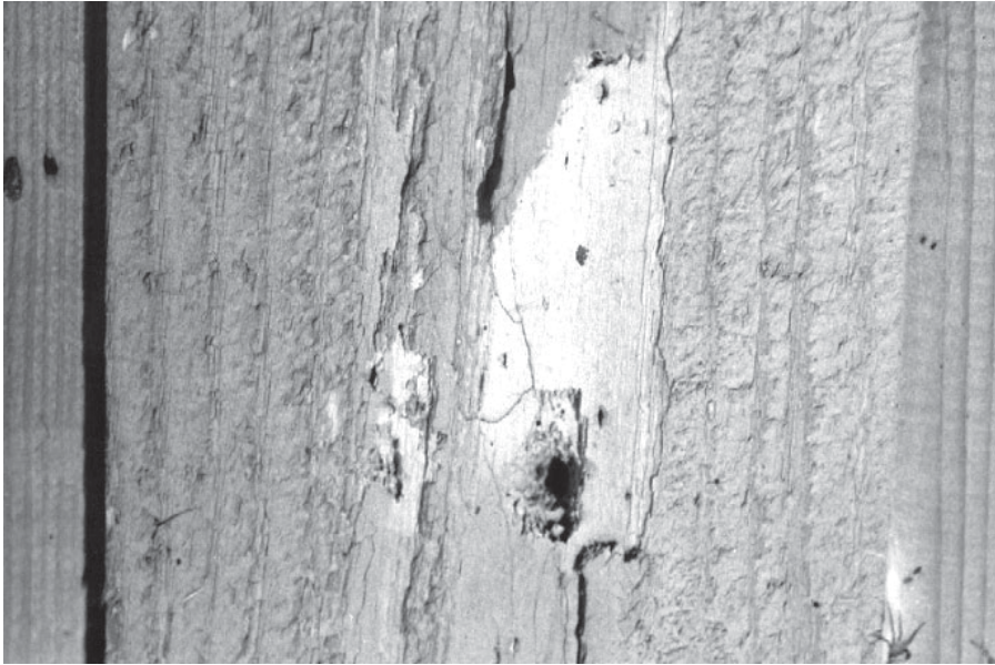
Figure 5—When growth rings separate from the rest of the wood, insects can enter a building's siding. Woodpeckers damage the siding when they feed on the insects.
